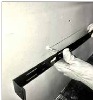
Figure 4.5 Installing Anchors in Hollow Wall
