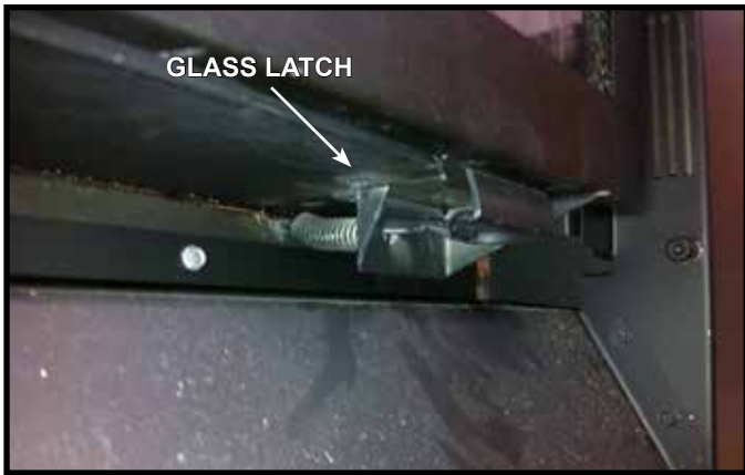
4.6 Glass Latch Detail - Exterior Side
