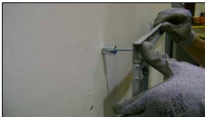
Figure 4.11 Installing Anchors in Hollow Wall
